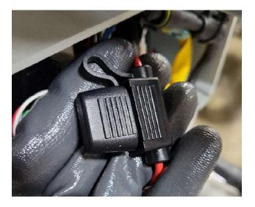
4. Identify if the fuse is blown. Sometimes this can be hard visually. If you are unsure, a multimeter continuity test would tell us for sure.
