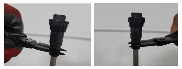
Step 8: Slide the rubber cover back over the connector body
